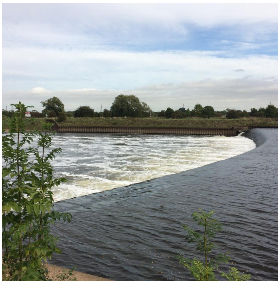
The River Trent at Cromwell Weir
