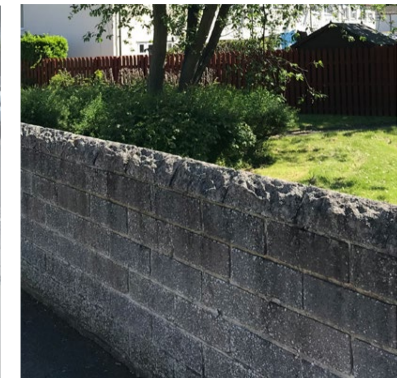
boundary wall repairs
