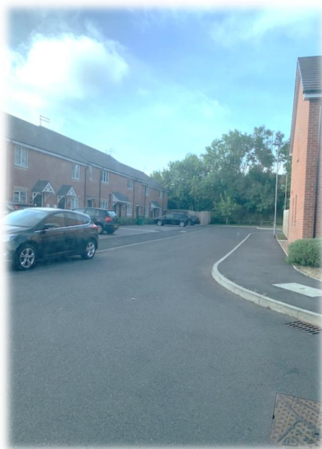
Figure 15: View of the development
