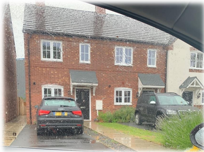
Figure 5: View of boundary separation between dwellings and their respective parking spaces
