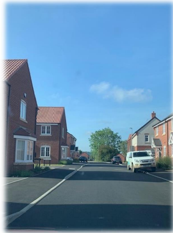
Figure 13: View down the central road running through the development
