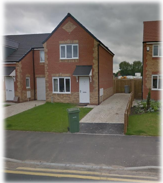
Figure 32: View of narrow driveway with bin blocking access
