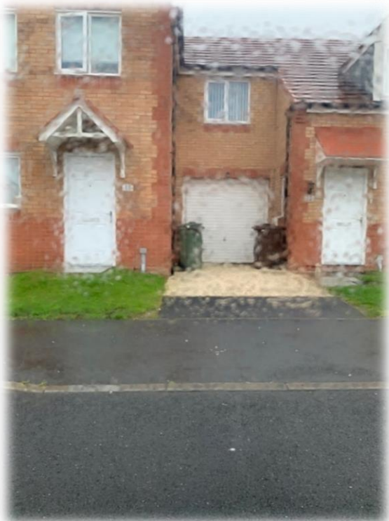
Figure 31: View of parking space being used to store bins
