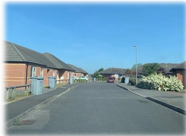
Figure 2: View of Development from Chewton Close
