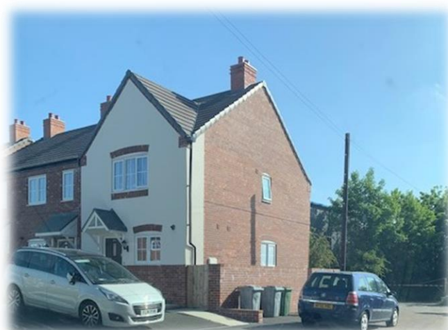
Figure 3: View of the only car parked on the road at the development
