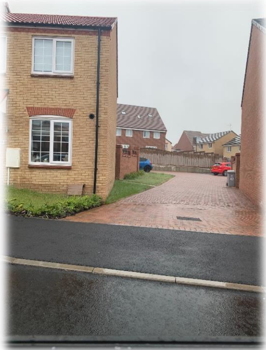
Figure 23: View of underused parking court adjacent to on street parking in Figure 22
