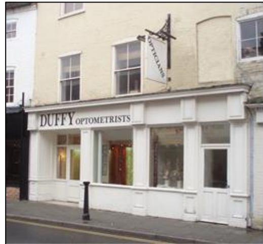
Figure 15: A new timber shopfront has been inserted into this building, replacing a poorly designed aluminium shopfront.
