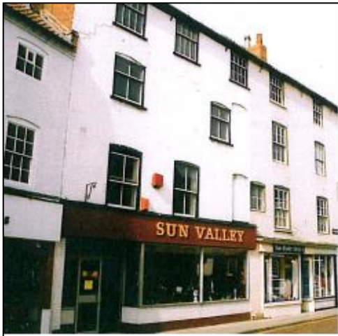
Figure 15: A new timber shopfront has been inserted into this building, replacing a poorly designed aluminium shopfront.
