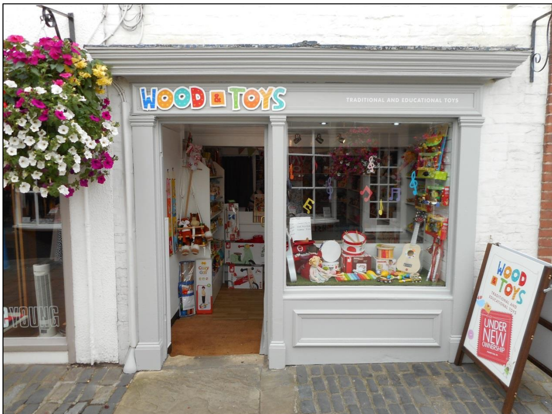
Figure 11: A shopfront painted off-white.
