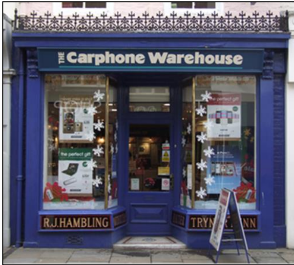
Figure 26: A national retailer occupies a listed shop where the original signage along the stallriser is retained.
