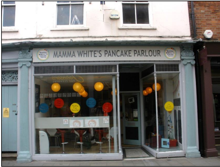
Figure 3: An example of an early 19 th century shopfront with later glazing.
