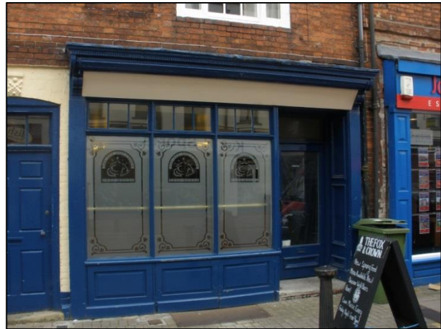
Figure 1: This shopfront was successfully altered as part of the conversion of this building into a public house. The removal of the Dutch blind and the insertion of a deeper panelled stallriser, along with mullions and transoms, gives a more successful shopfront design.
