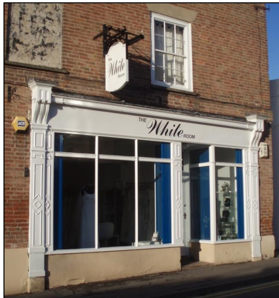
Figure 17: A well detailed timber shopfront where colours have been kept very simple to give a striking effect.
