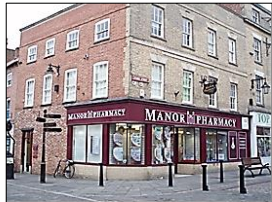
Figure 27: The overlarge fascia sign used to cut through the first floor windows, destroying their proportions. The shopfront and fascia signage has been replaced with a more sympathetic, traditionally detailed design which has restored the windows to the first floor.
