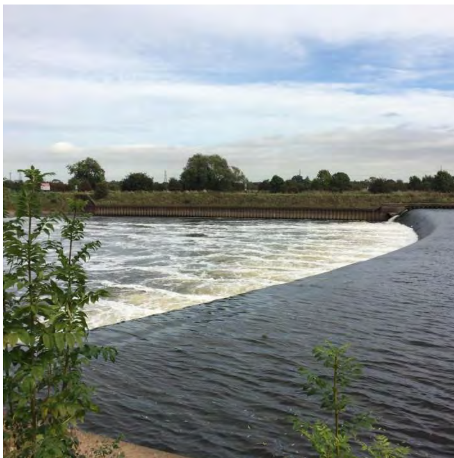
The River Trent at Cromwell Weir
