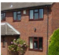
Brown windowframes and weather boarding.
