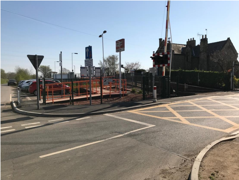
Fiskerton Station Level Crossing
