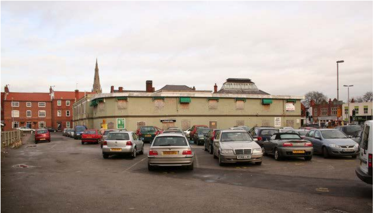
The rear car park in early 2000s.
